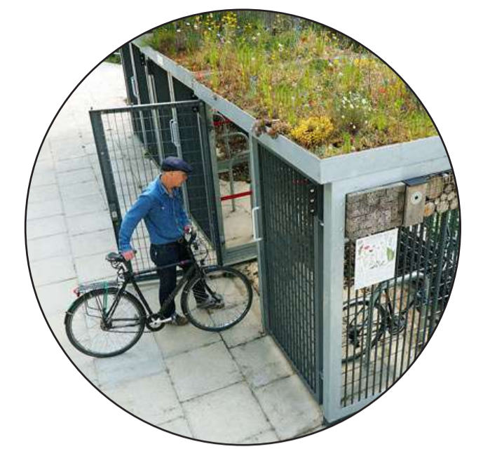
Cycle shelter with green roof
