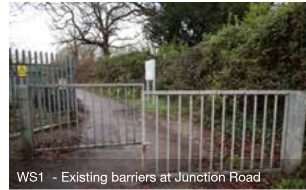
WS1 - Existing barriers at Junction Road
