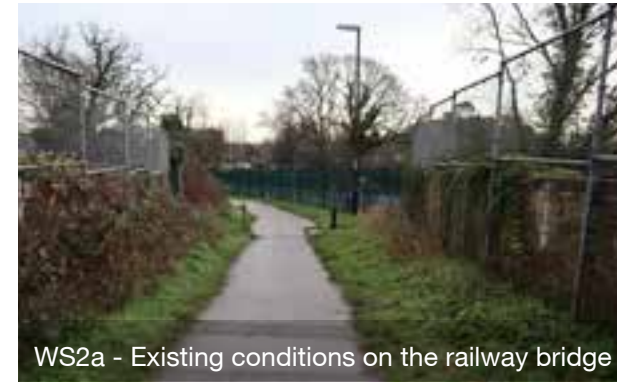
WS2a - Existing conditions on the railway bridge
